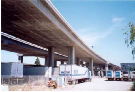
Figure 7. I-880 testbed bridge (author photo).
