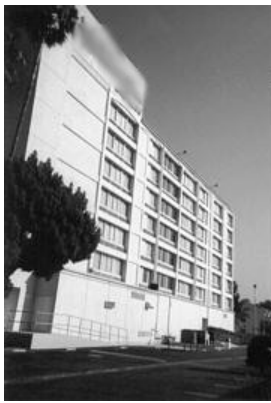
Figure 4. Van Nuys testbed building in 2000 (author photo).
