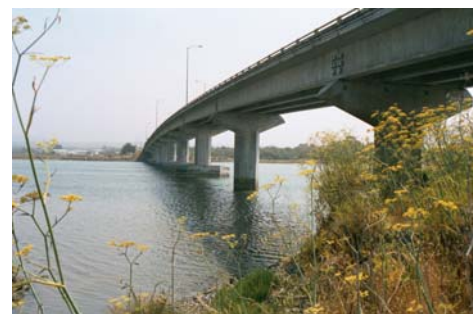
Figure 6. Humboldt Bay Bridge (G. Deierlein photo).
