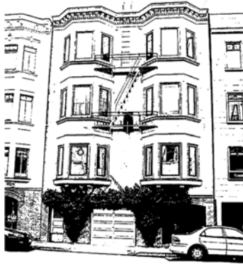
Figure 1. Index buildings. Four older, soft-story, woodframe, multifamily dwellings representing a realistic range of performance of buildings of this class in San Francisco: (1) corner, 3 story, no interior walls at garage level, one street facade \geq 80\% open at ground floor; (2) corner, 4 story, both street facades \geq 50\% open at ground floor; (3) mid-block, 4 story, pre-WWII, neighbors on both sides; (4) mid-block, 3 story, post-1950, neighbors on both sides. Square footage is 3,600, 5,800, 2,300, and 1,800 sf, respectively.
