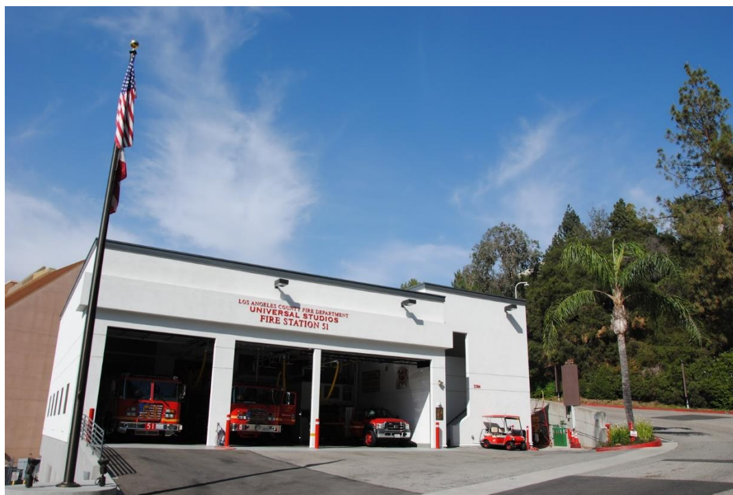
Figure 1. Earthquake early warning can automatically open fire station bay doors and sound an audible alarm through the fire station public address system, two-way radio system, or both (image: anonymous, CC-BY-SA 4.0)
