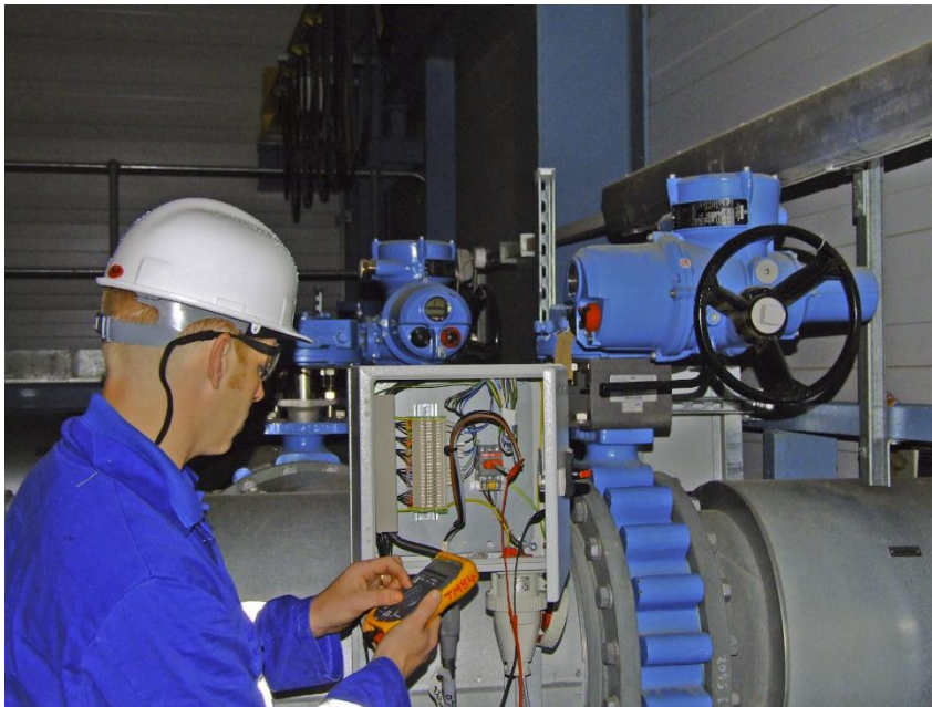
Figure 1. Earthquake early warning can automatically close or open valves, start or stop electrical equipment, open doors, sound alarms, or shut off power to protect water and wastewater systems. (Image: Khepster, 2008, Creative Commons Attribution 3.0)
