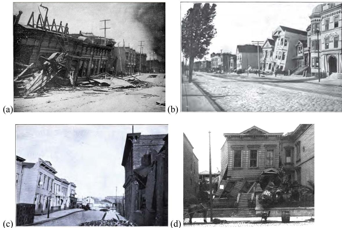
**Figure 2.** Collapses of large midblock woodframe building in the 1906 San Francisco earthquake: (a) Valencia St. Hotel (Pierce 1906), (b) Howard St (Gilbert et al. 1907), (c) Dore St. between Bryant and Brannan (Gilbert et al. 1907), (d) unknown location, where collapse is associated with “cripple-wall and shear failure” (Tobriner 2006)
