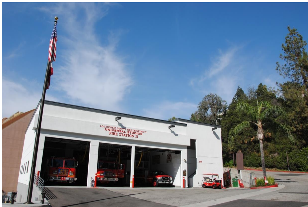
Figure 1. Earthquake early warning can automatically open fire station bay doors and sound an audible alarm through the fire station public address system, two-way radio system, or both (image: anonymous, CC-BY-SA 4.0)
