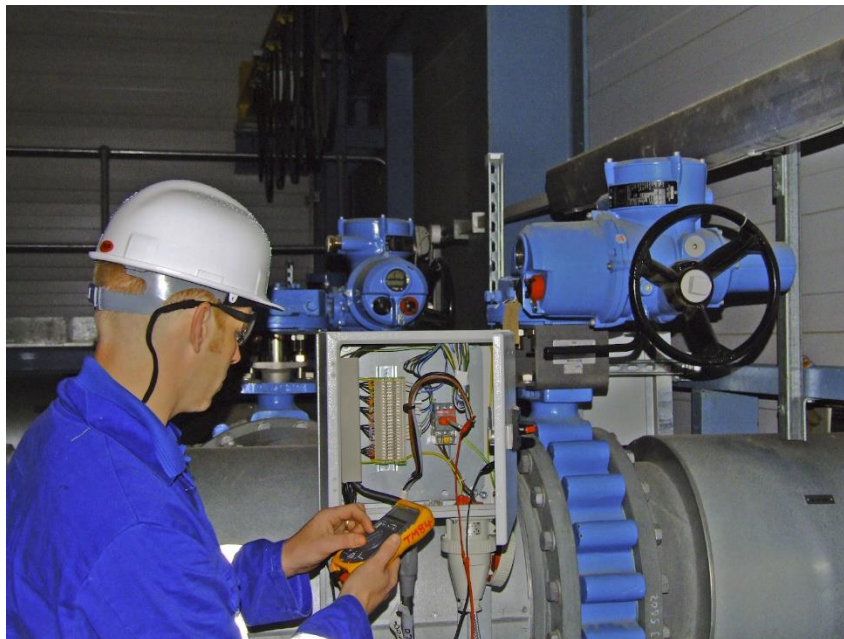
Figure 7. Earthquake early warning can automatically close or open valves, start or stop electrical equipment, open doors, sound alarms, or shut off power to protect water and wastewater systems. (Image: Khepster, 2008, Creative Commons Attribution 3.0)
